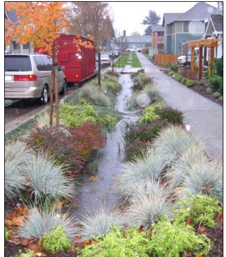
A bioswale collects and infiltrates stormwater rather than directing it to a drainpipe, reducing run-off and improving water quality.
