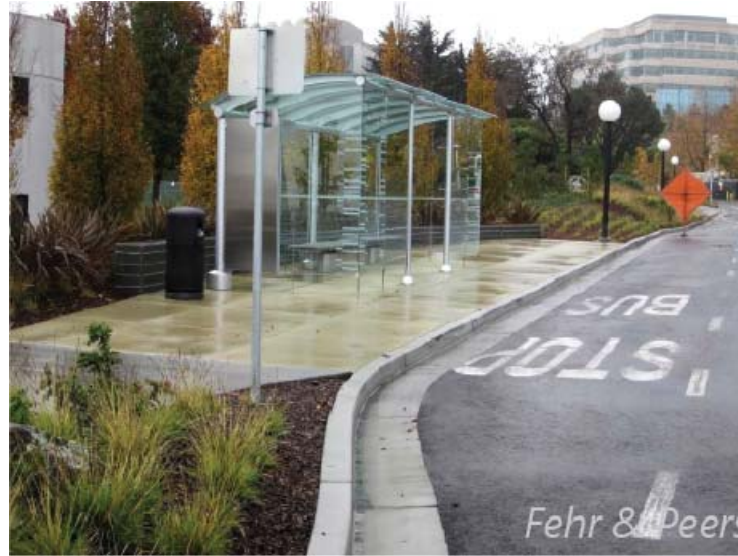
Bus shelter with passenger amenities.
