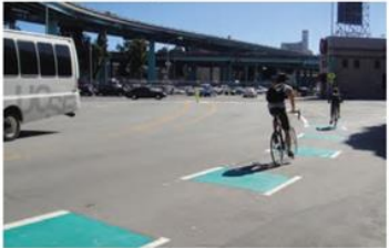
2. Green striping on a Bike Lane
