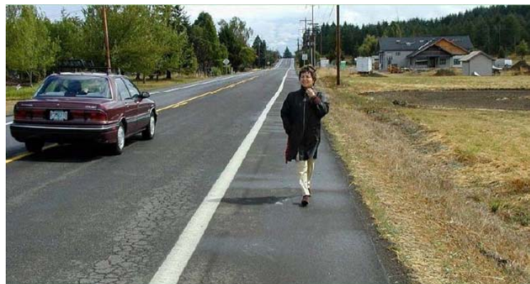
Paved shoulders (6 feet preferred) provide safe walking areas for pedestrians along Rural Connectors and can also improve space for cyclists.
