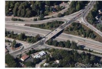
9. HWY1 / Rio Del Mar Diamond Interchange
