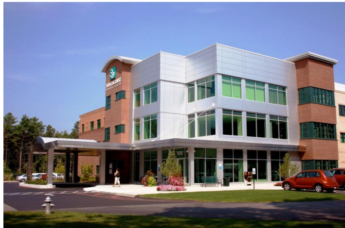
Mixed-use development along Soquel Drive (top) complements new medical uses (bottom) to enhance a dynamic employment center
