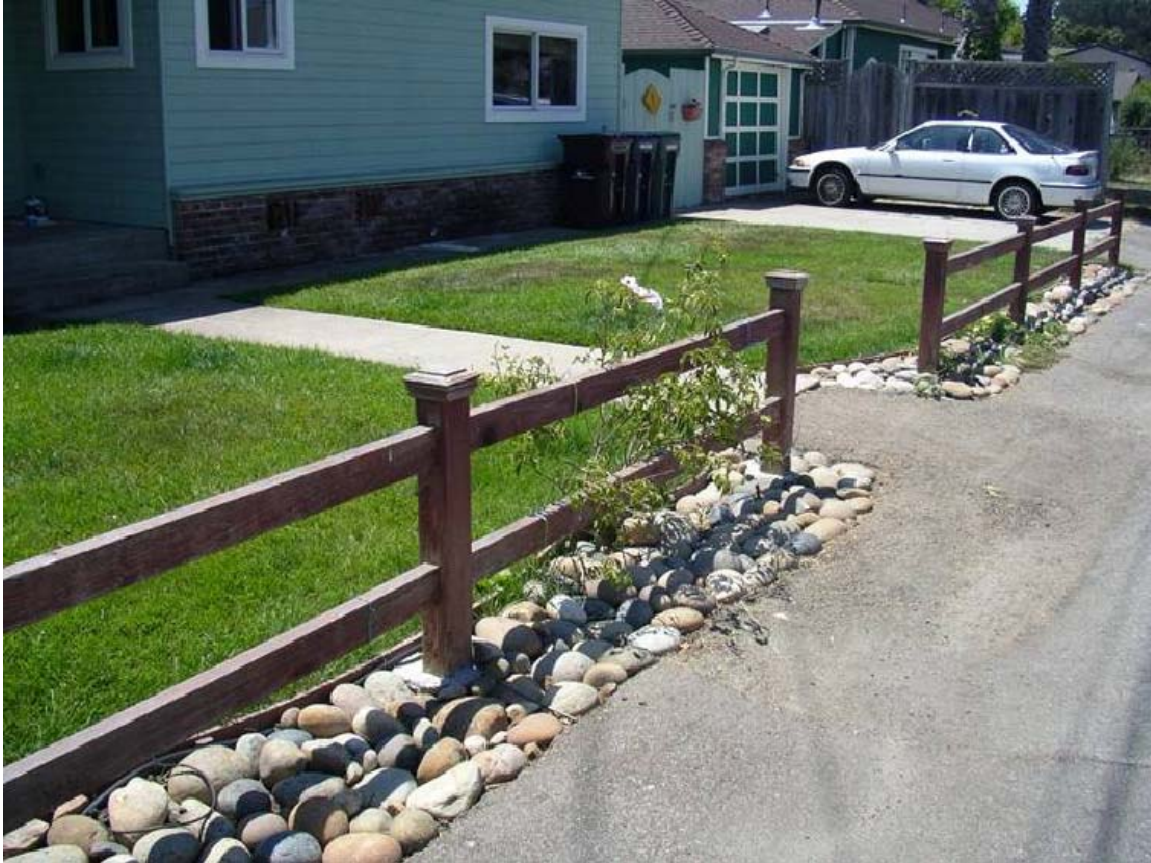
Porous Drainage Treatment Helps to Infiltrate Runoff
