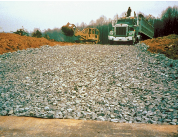
Picture 7. Rocked Construction Entrance.
