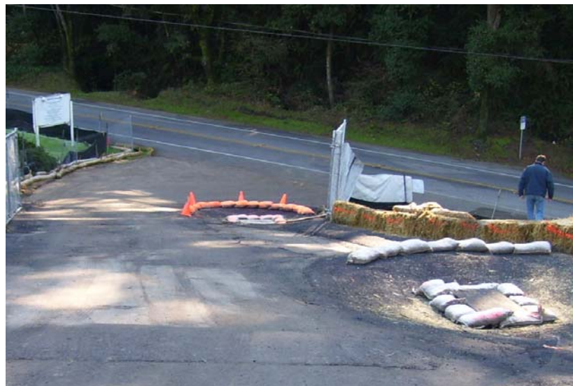
Picture 6. Use of gravel bags for protection of drainage inlets.
