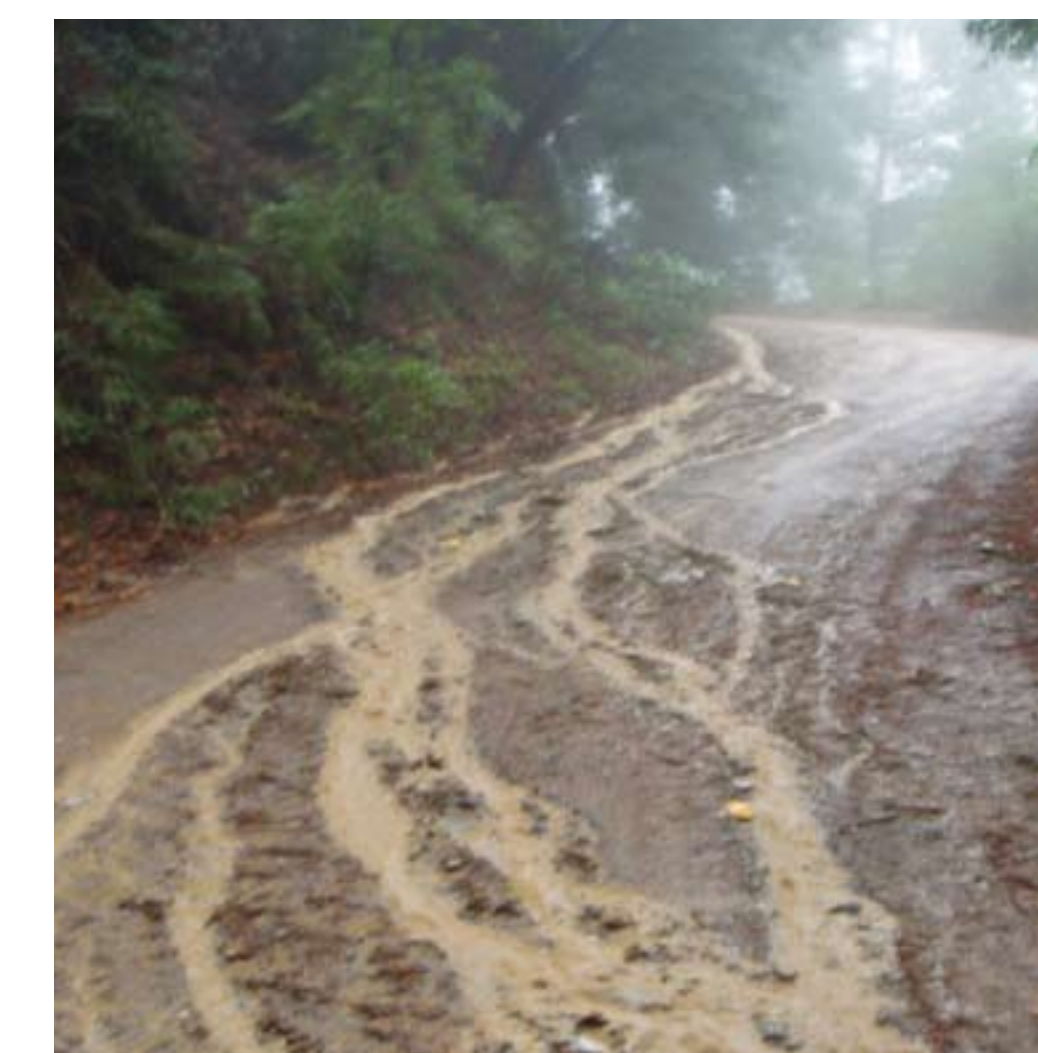
PROPER DRAINAGE ON DIRT ROADS CAN PREVENT EROSION AND REDUCE MAINTENANCE COSTS
