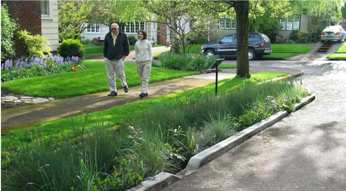
Example of a Local Neighborhood Street Storm Water Drainage Solution in Portland, Oregon
