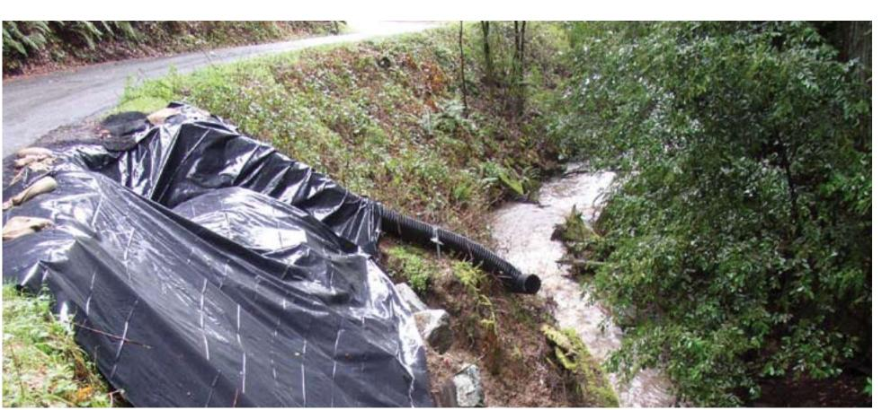
THIS ROAD SLIP OUT DELIVERS SEDIMENTS DIRECTLY TO THE STREAM
