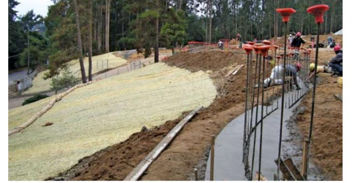
**EROSION CONTROL METHODS INCLUDE BLANKETS, WATTLES** (ROLLS), MULCHING AND SEEDING
