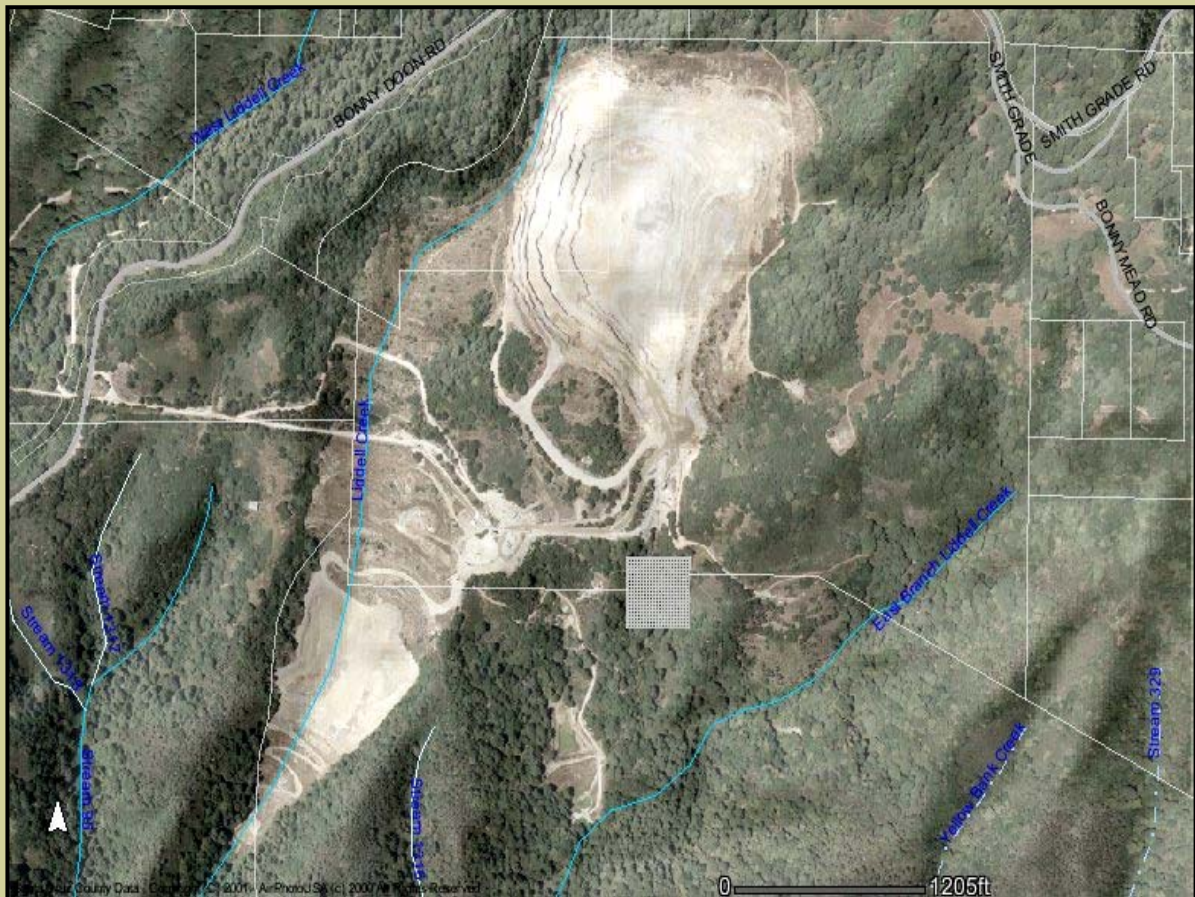
This aerial photograph shows the Bonny Doon Limestone Quarry. Source: County of Santa Cruz, 2007.
