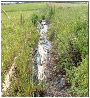
Photograph 14. View of black plastic-lined ditch along northeastern Project boundary. Ditch drains southwest.
